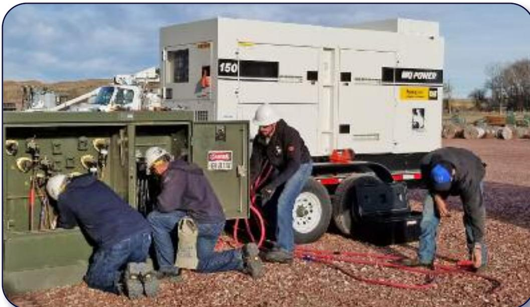
The Wyrulec crew hooked up the new generator for a trial run to power the headquarters building.
